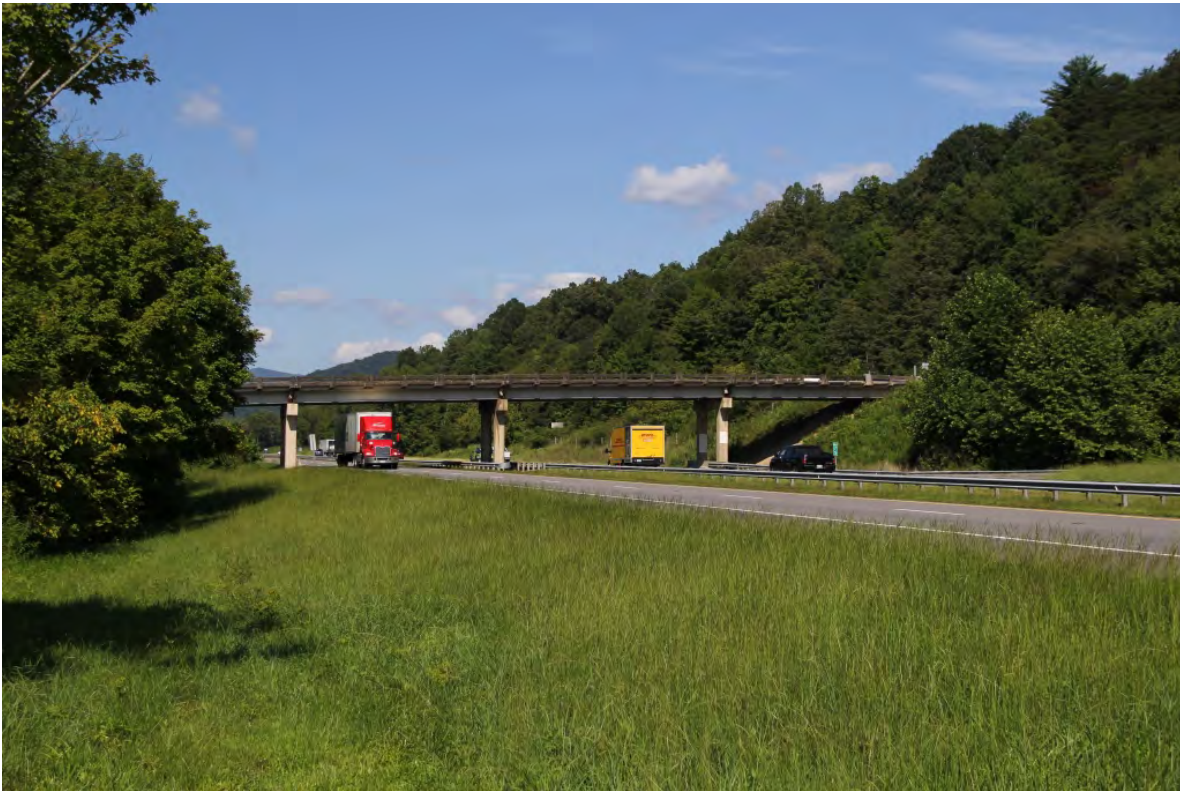
Bridge No. 84 on SR 1234 (Parker Padgett Road) over I-40, Exit 75, view to west
