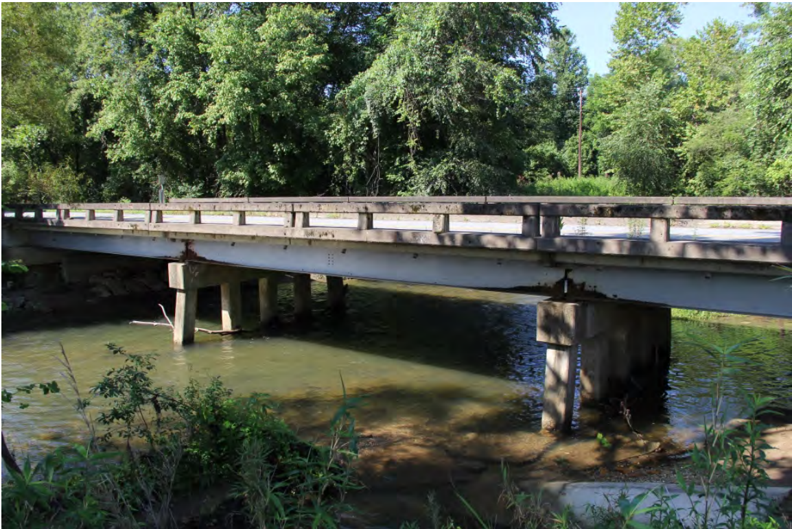
Bridge No. 142, east side, oblique view to southwest
