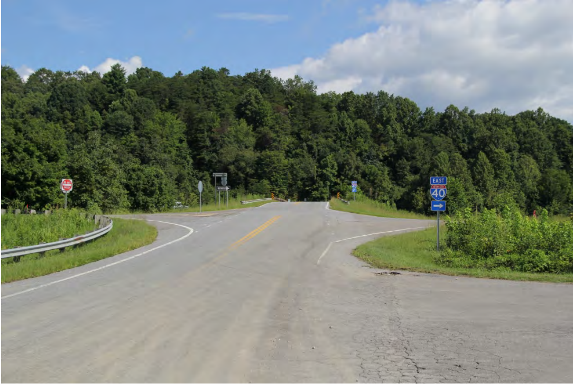
Bridge No. 84 (Exit 75), view to north along SR 1234 (Parker Padgett Road)
