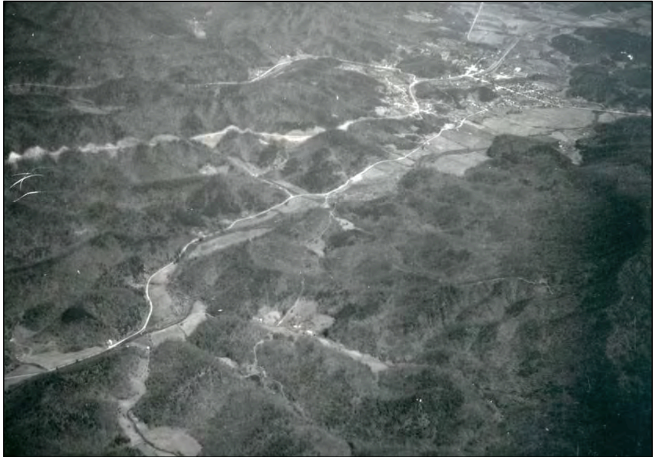
I-40 Construction, WSW from Old Fort along Catawba River, April 6, 1958, Bingham Aerial Photo [E243-5, North Carolina Collection, Pack Memorial Library, Asheville, NC]
