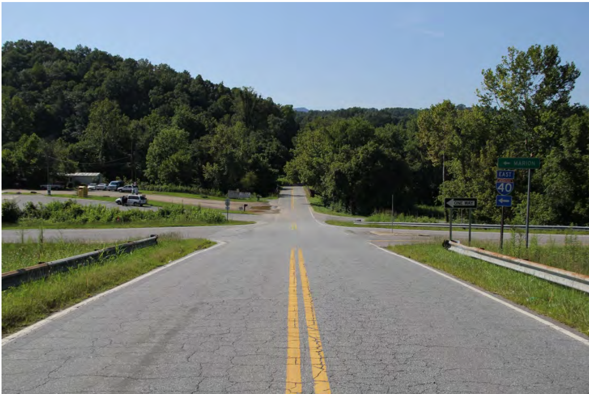
Parker Padgett Road (SR 1234), view south from Exit 75 toward Bridge No. 142
