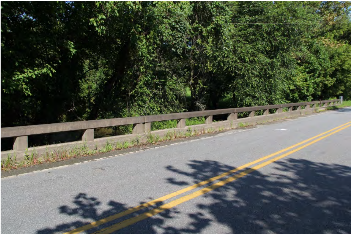
Bridge No. 142, west railing, view to northwest
