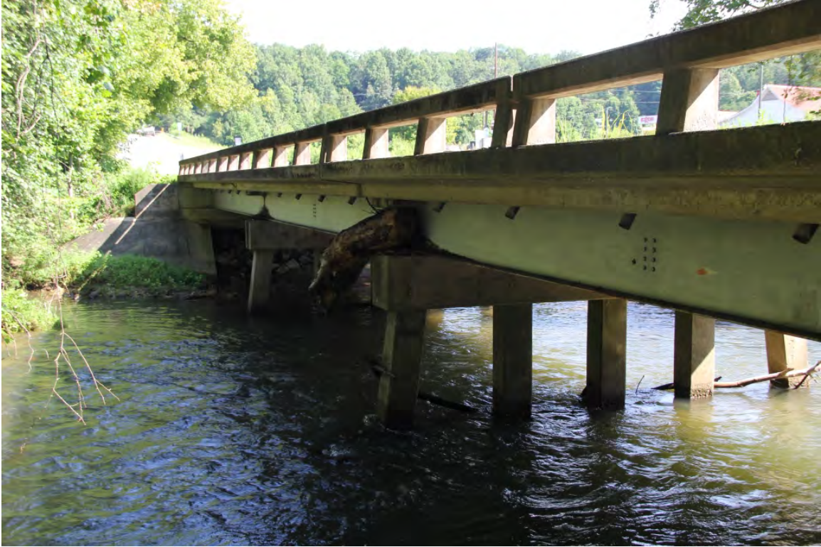
Bridge No. 142, west side, oblique view to northeast
