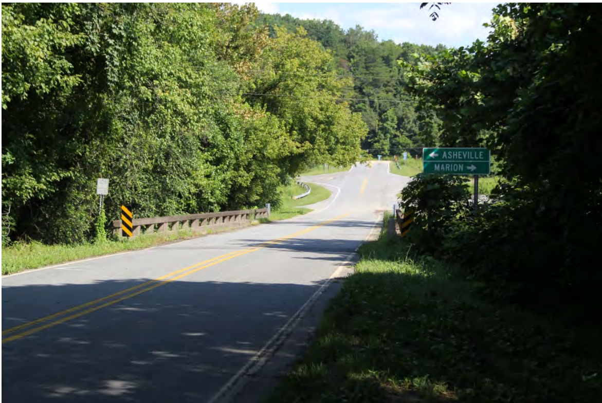
Bridge No. 142 over Catawba River, view to north along SR 1234 (Parker Padgett Road)
