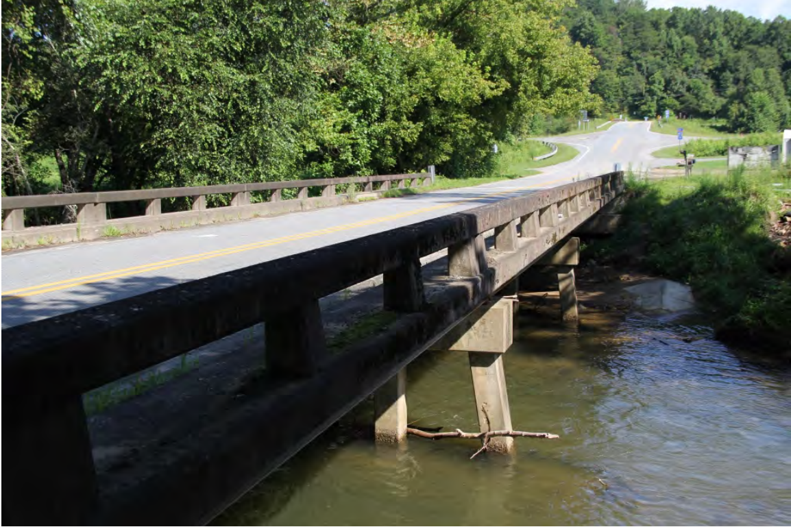
Bridge No. 142, east side, oblique view to north
